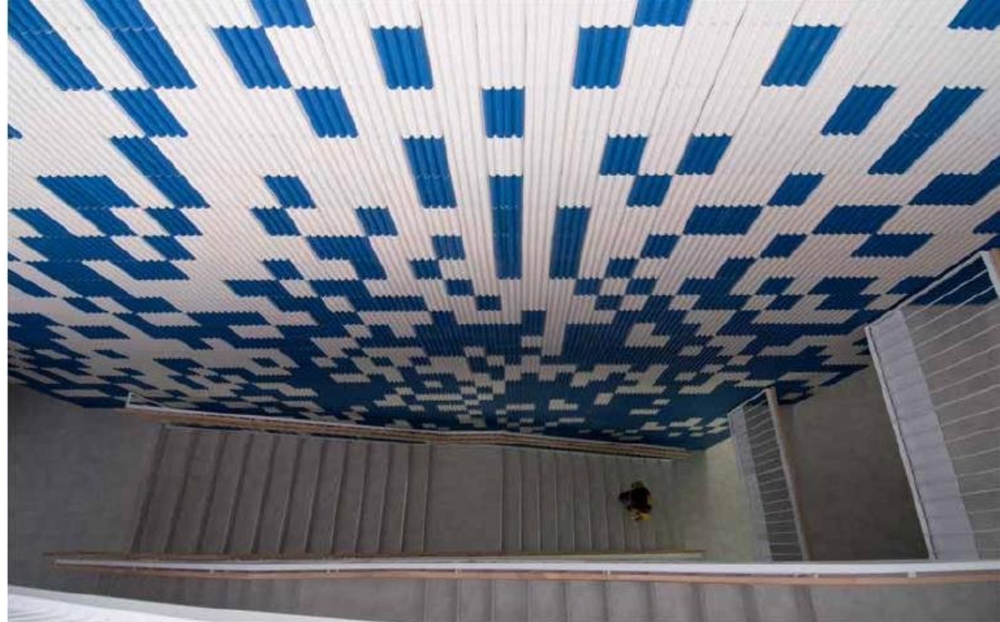
Los Llanos Adult Education Center in Albacete by Matos-Castillo Arquitectos. Exterior skirting and lobby clad in blue and white glazed undulating stoneware tiles.
