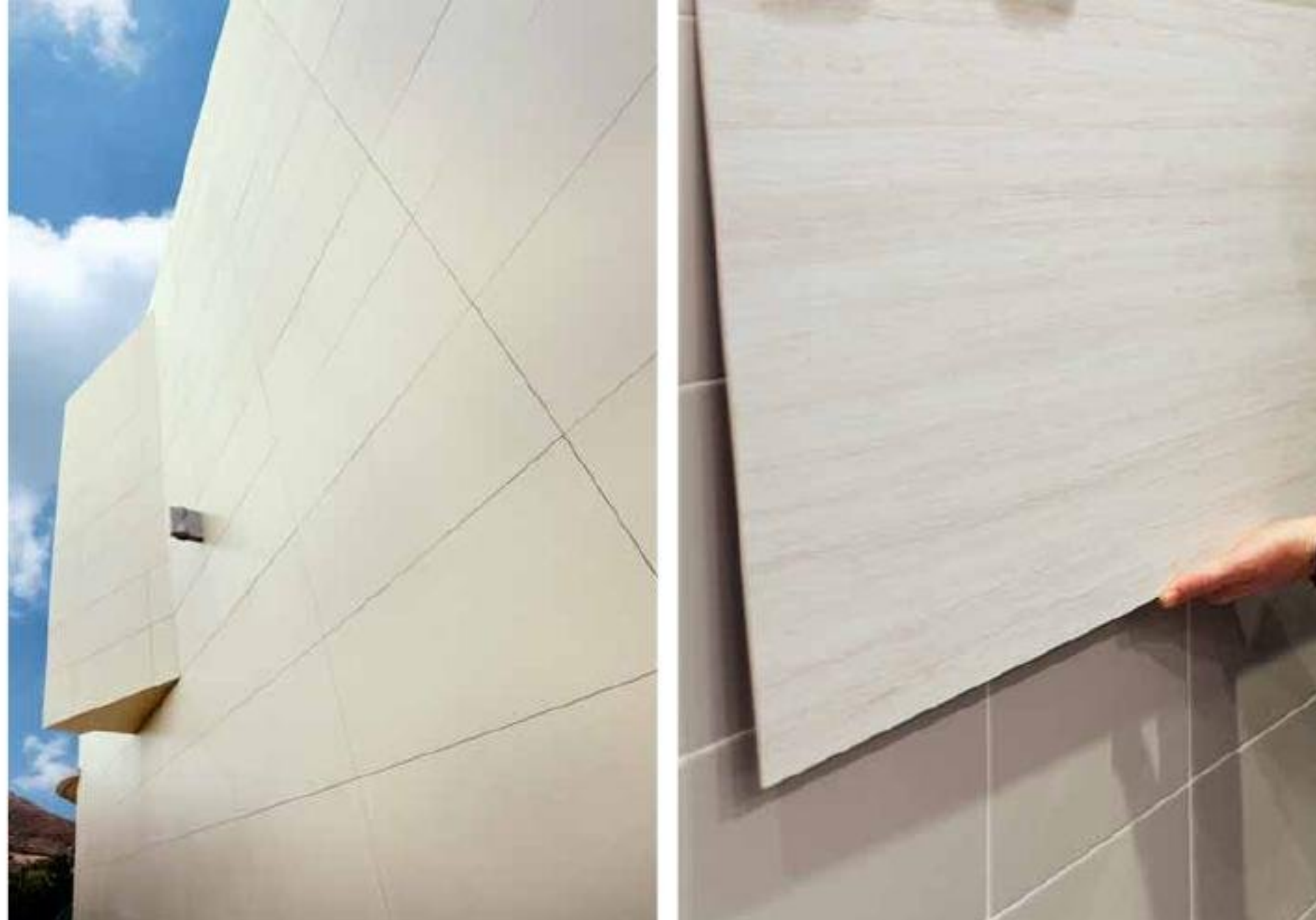
Renovation of a single family house in Murcia. Using minimum thickness ceramic tiles made it possible to renovate both the exterior and the interior rooms, without having to remove the existing coverings, thereby avoiding demolition, noise and mess. Coverlam series, 3.5 mm (.1 inch) thick porcelain.
