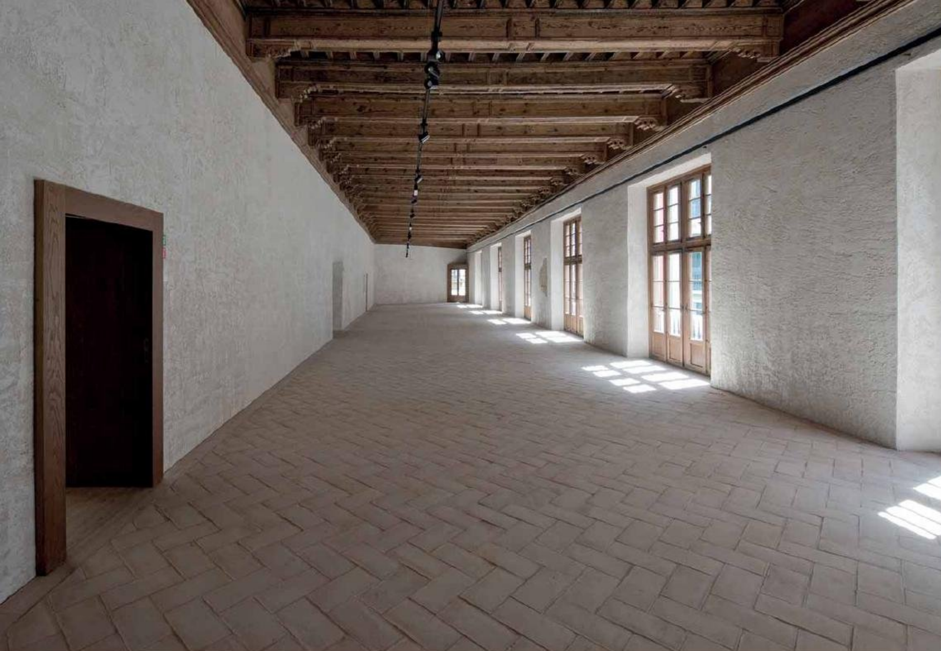
In the renovation of the Casa del Condestable (Pamplona) by Tabuenca & Leache the custom-made terracotta tiles used are the link between the past and the present.
