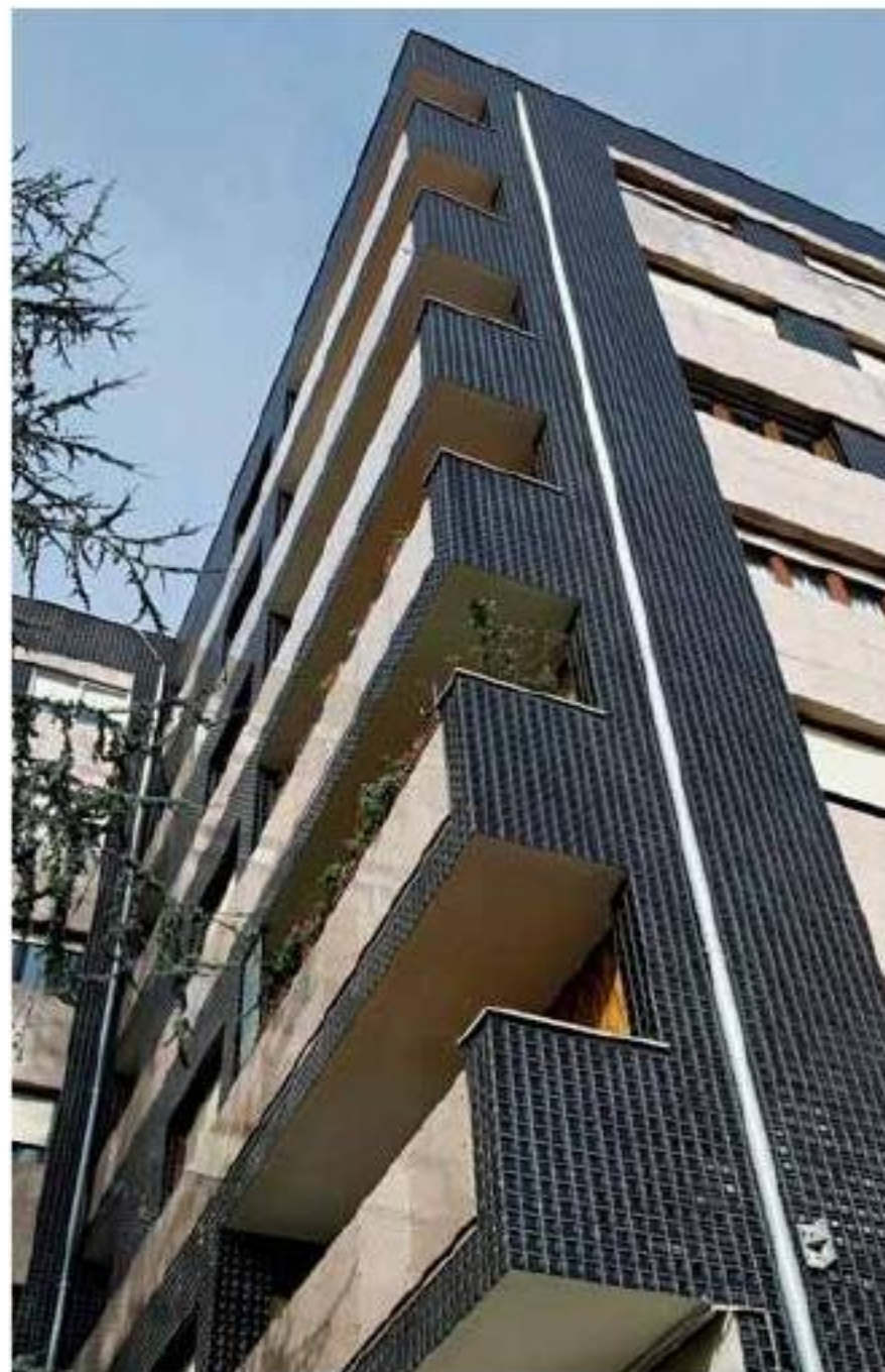
Renovation of an apartment block in Leioa (Vizcaya) where the owners wanted to retain the use of ceramic tiles on the facade but with a modern yet timeless design. The tiles are 10x10cm (4X4 inches) stoneware, suited to external use (Dune Cerámica, Black Infinity series - Emphasis Ceramics Collection).
