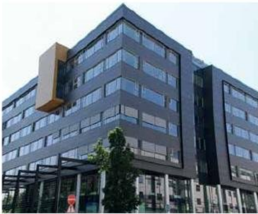
The use of TECHLAM® by Levantina on the facade of the Green House Building is what won it the sustainability category.
