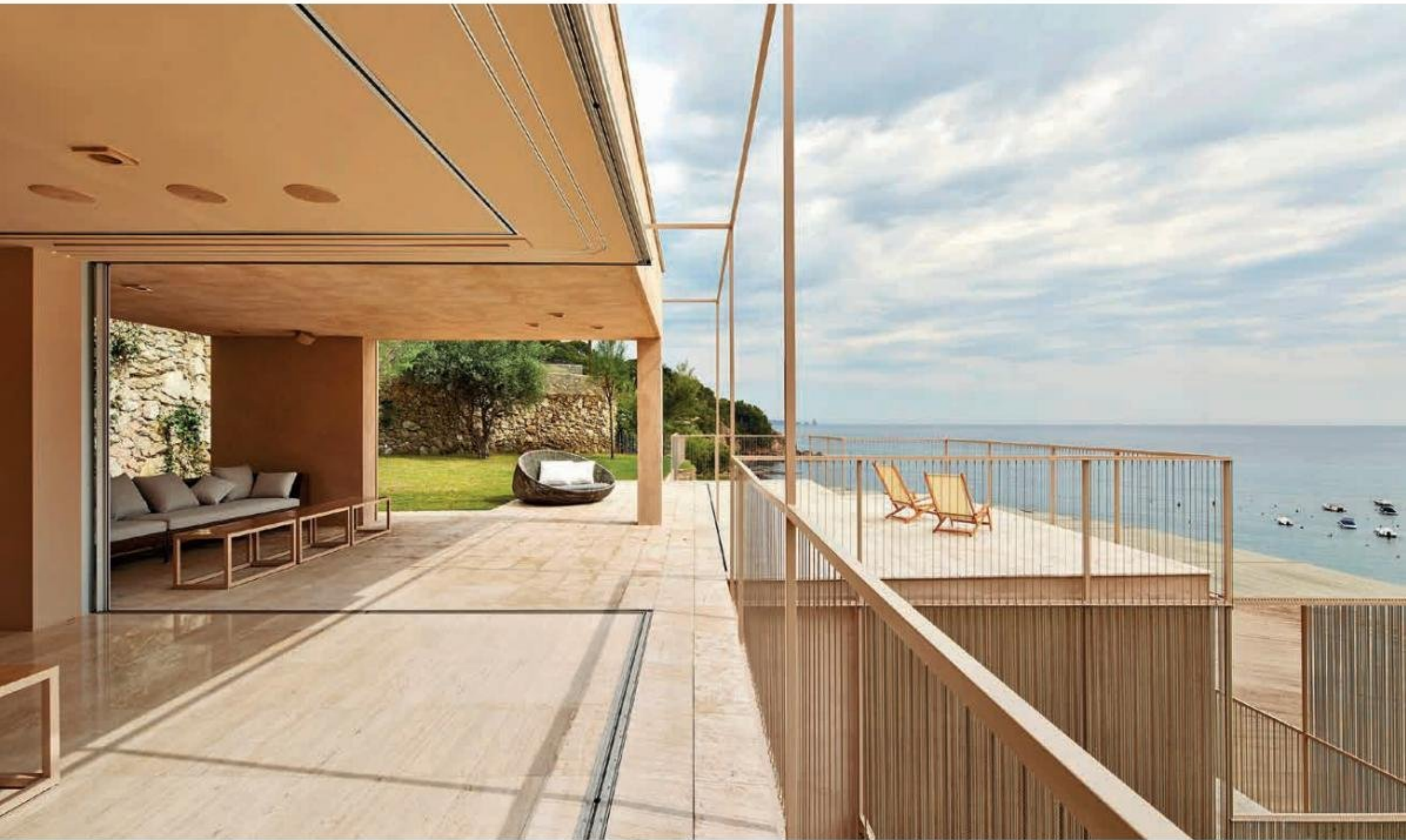
General view of Casa Andamio © Jose Hevia.
