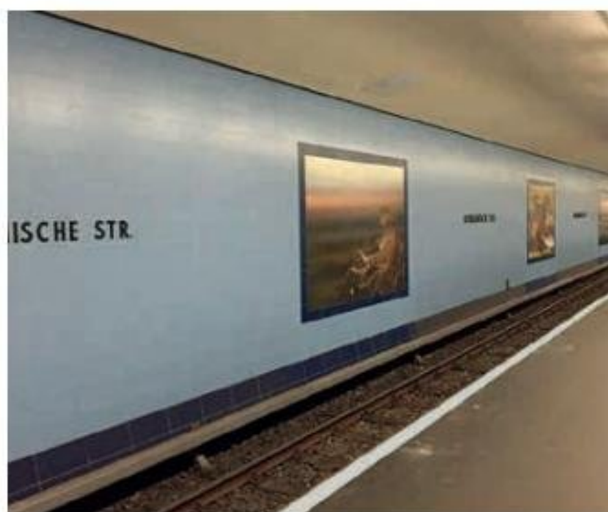
Station in the Berlin underground. Cladding in porcelain stoneware by Ceracasa Emotile.
