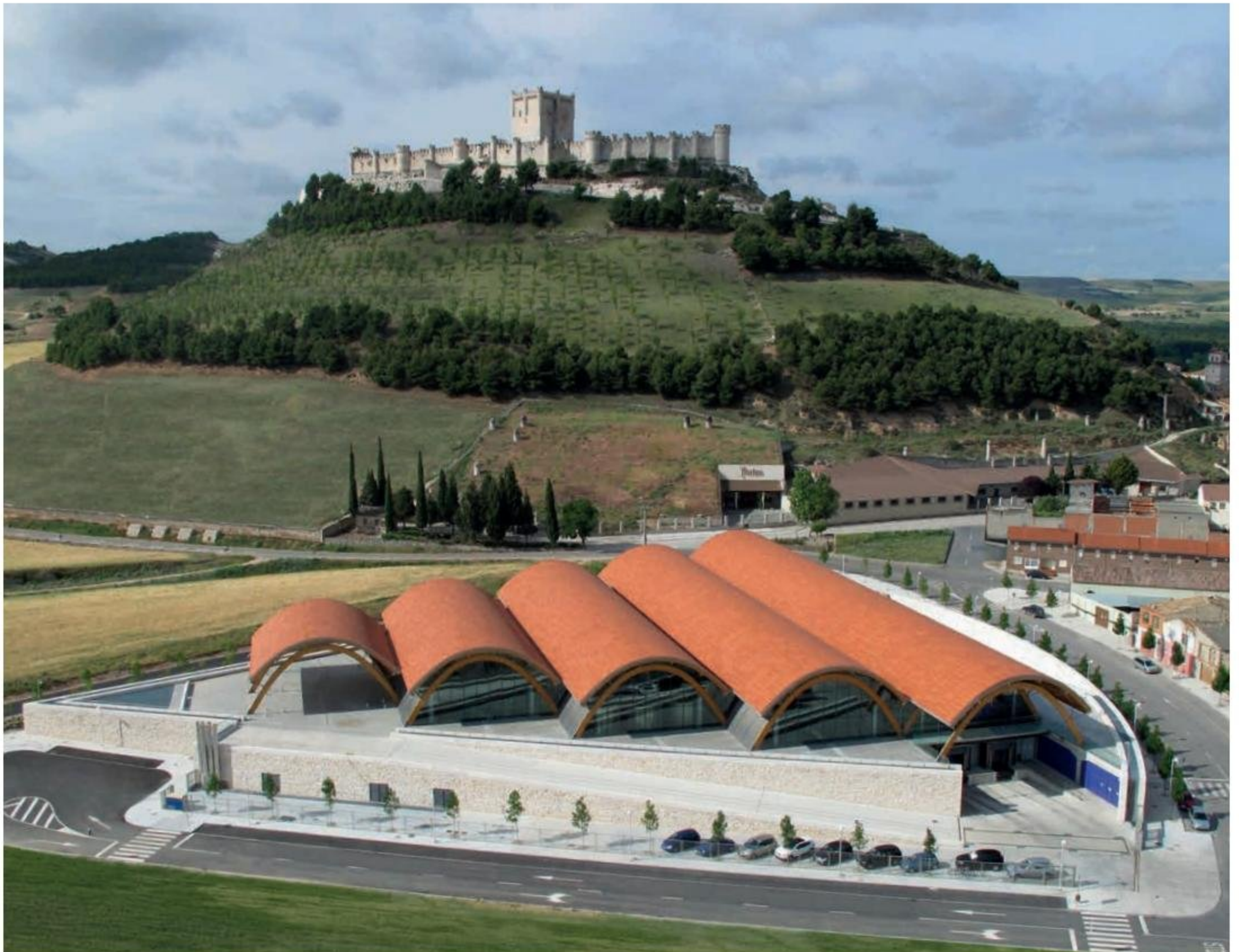
Ceramic tile roof at Bodegas Protos in Peñafiel, by architects Rogers Stirk + Alonso Balaguer asociados.
