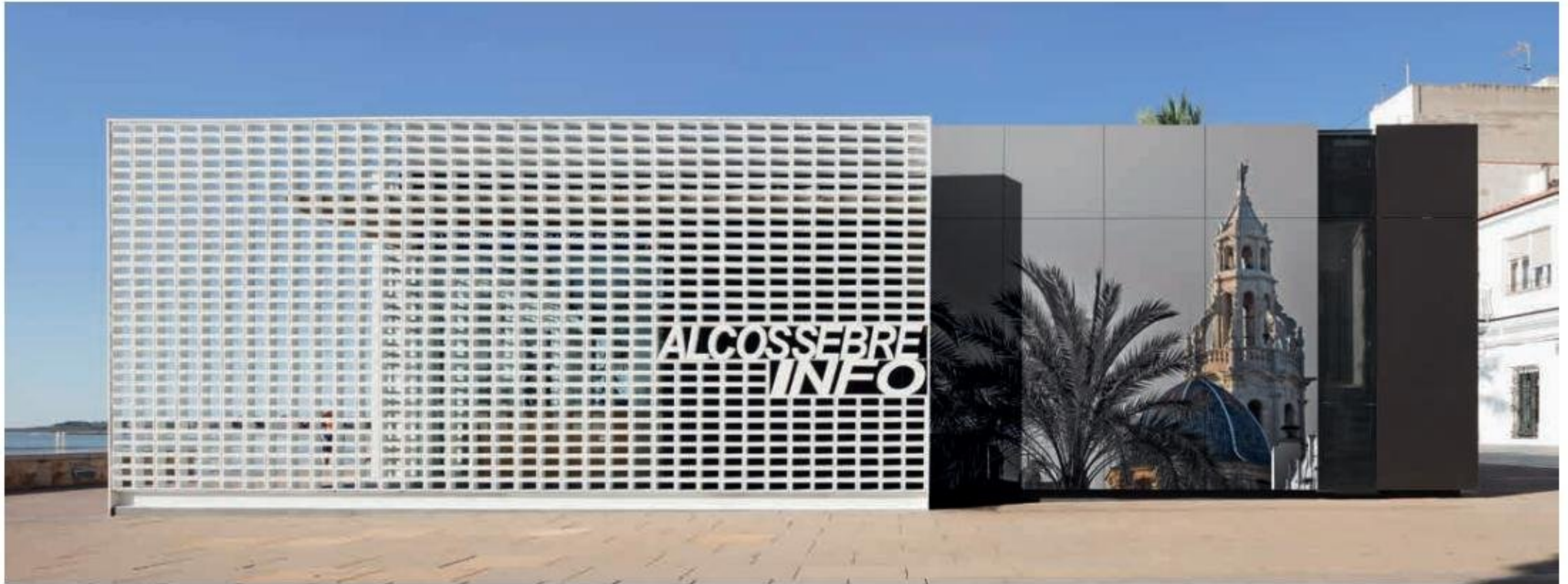
Urban intervention in Alcocebre by Sanahuja & Partners Ceramic finish by Grespania Coverlam using H&C TILES.
