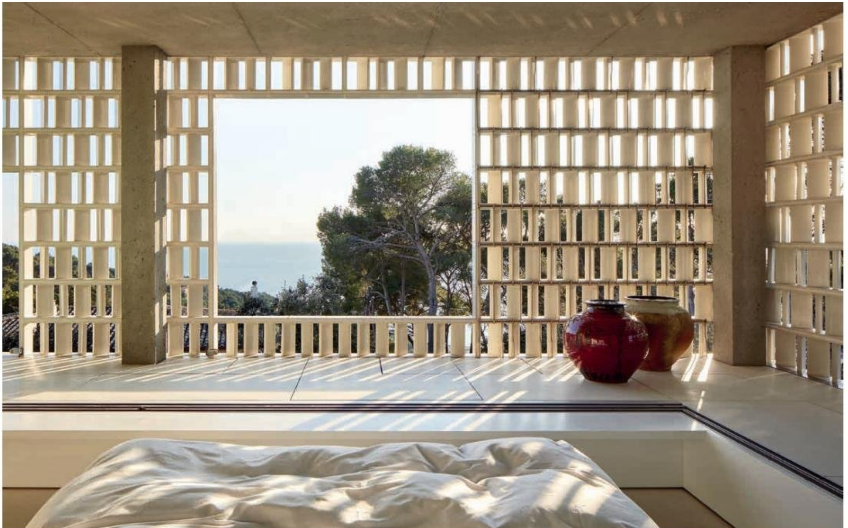
Controlling exposure to sunlight with 'broken' ceramic tiles. Casa Celosía (Lattice House) by Emiliano López Matas.
