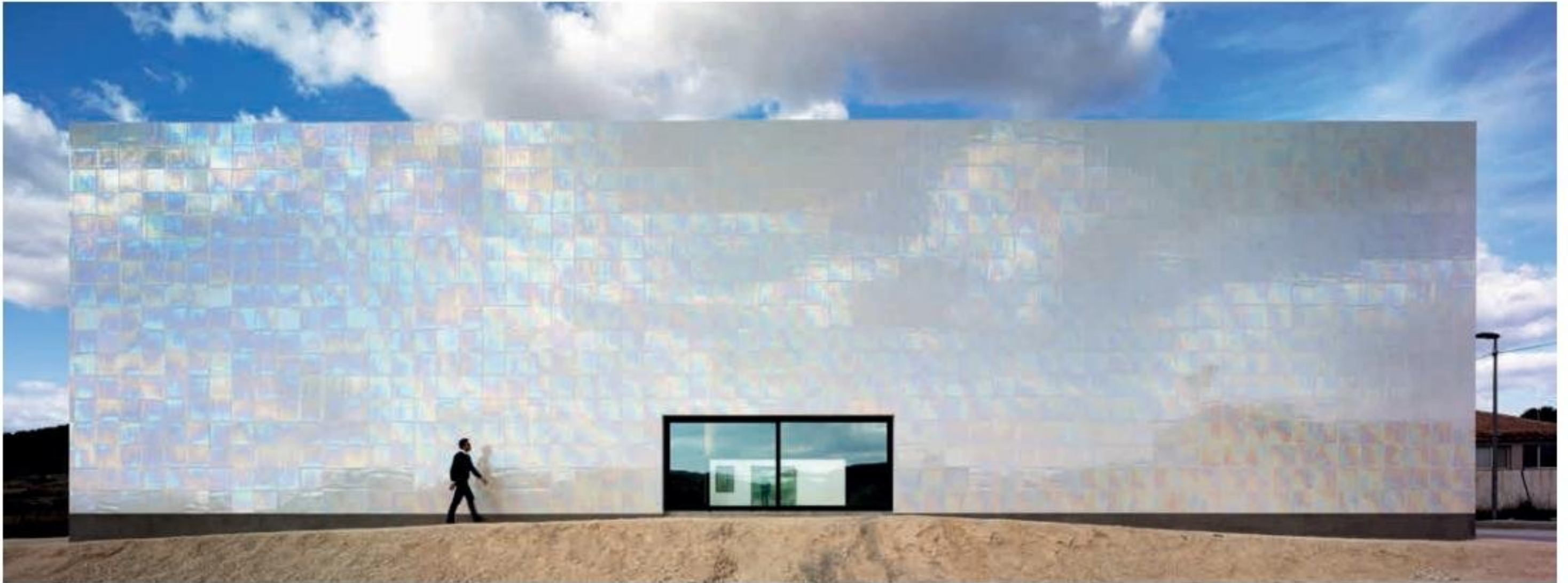
Pearlized ceramic facade. MUCA Building, by COR Arquitectura.
