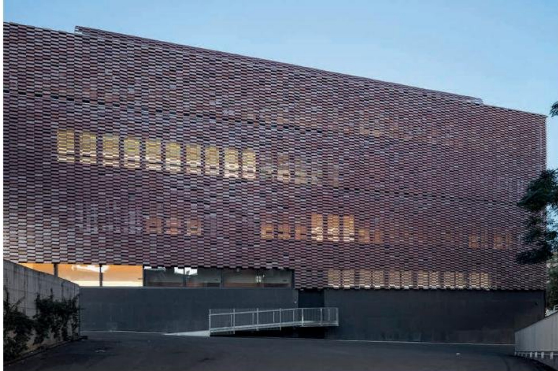
GRES ARAGÓN, Research center at the Hospital de la Santa Creu i Sant Pau, Barcelona - ventilated facades Series Faveker Collection.
