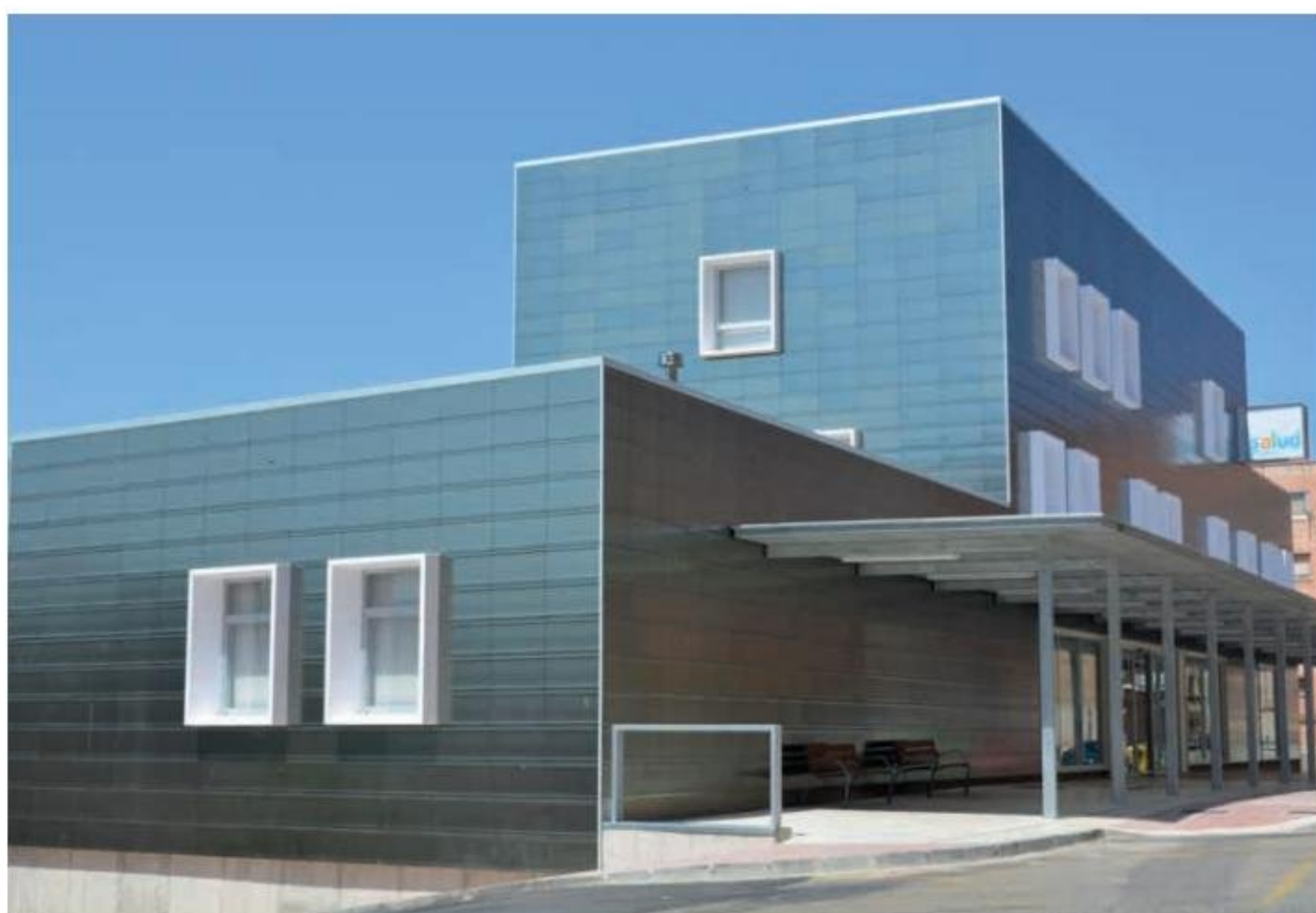
GRES ARAGÓN, Illueca Municipal Health Center- ventilated facades Series Faveker Collection.
