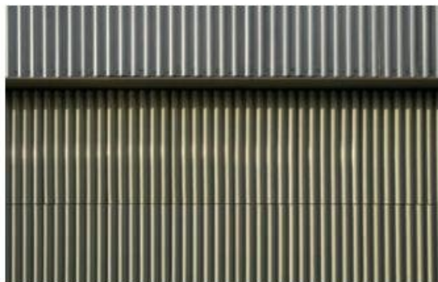
Runnymede College campus by architects Rojo / Fernández-Shaw. Awarded a special mention in the architecture category. Photographs: Luis Asín.
