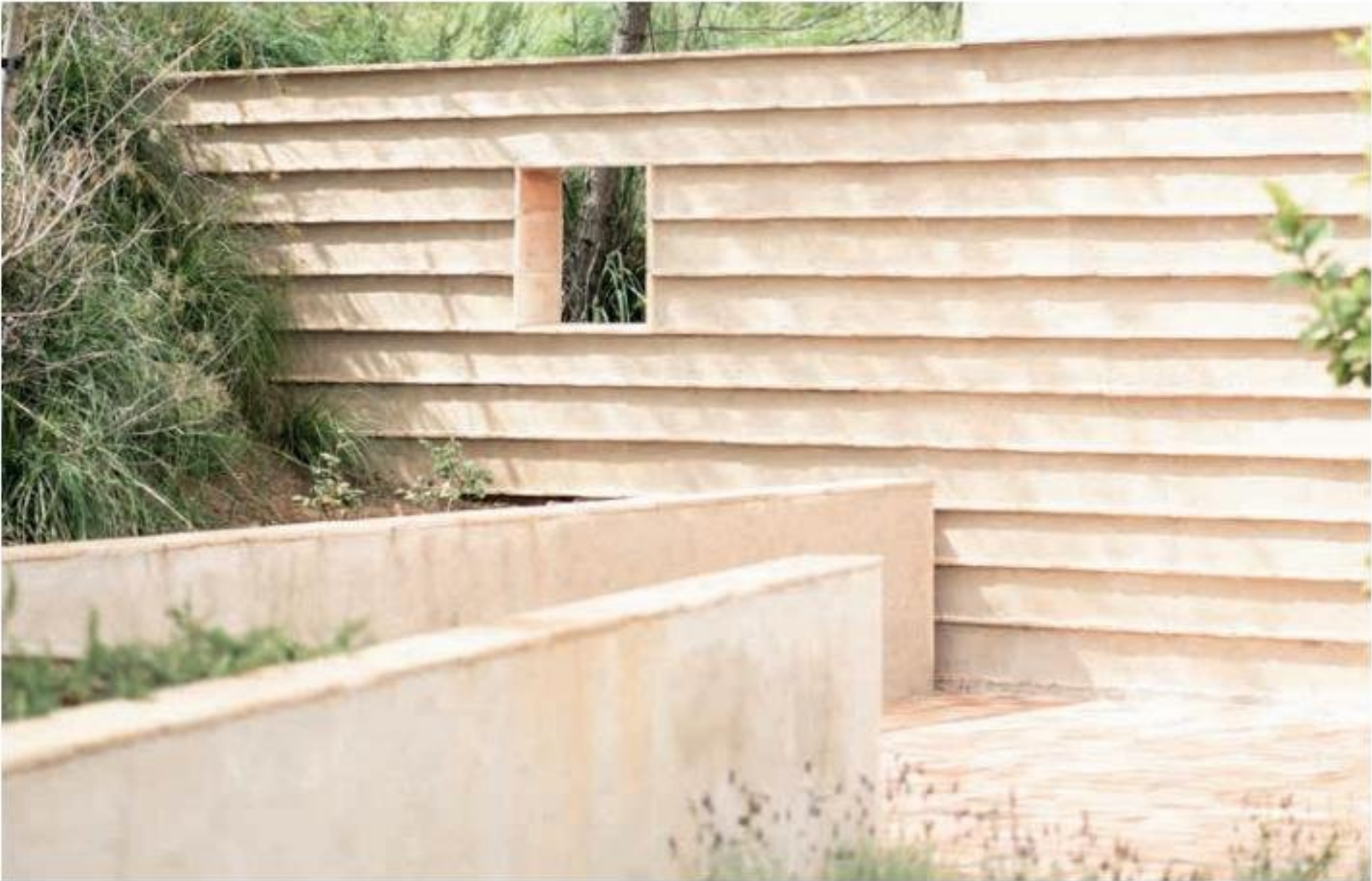
The outside of "Casa Ter" by Mesura. Photographs: Salva López & Mesura.
