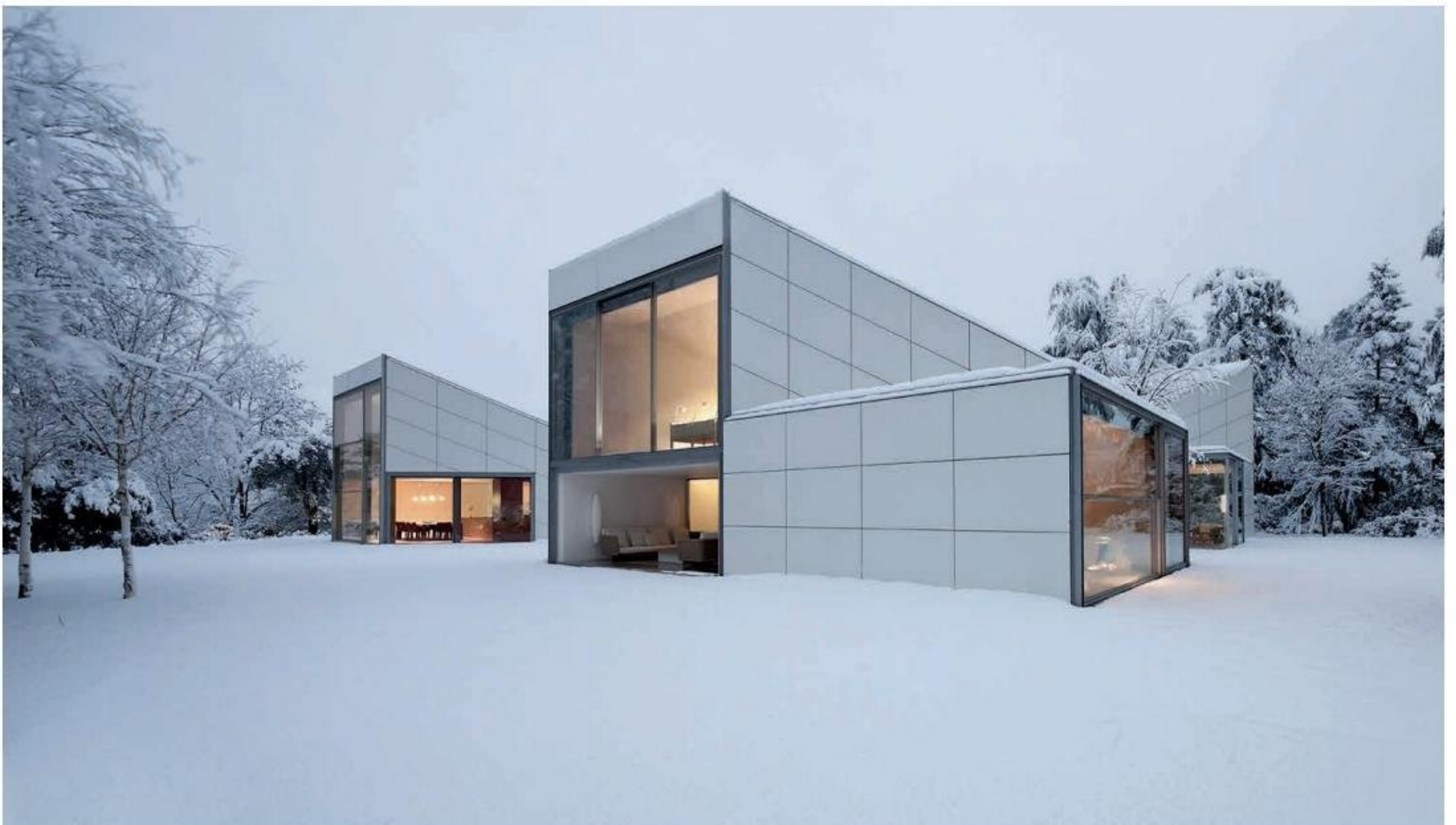
Casa AA by architects Carlos Ferrater & Xavier Martí, OAB (Barcelona). Built in 2011. Large-format slimline ceramic sheets by Saloni.
