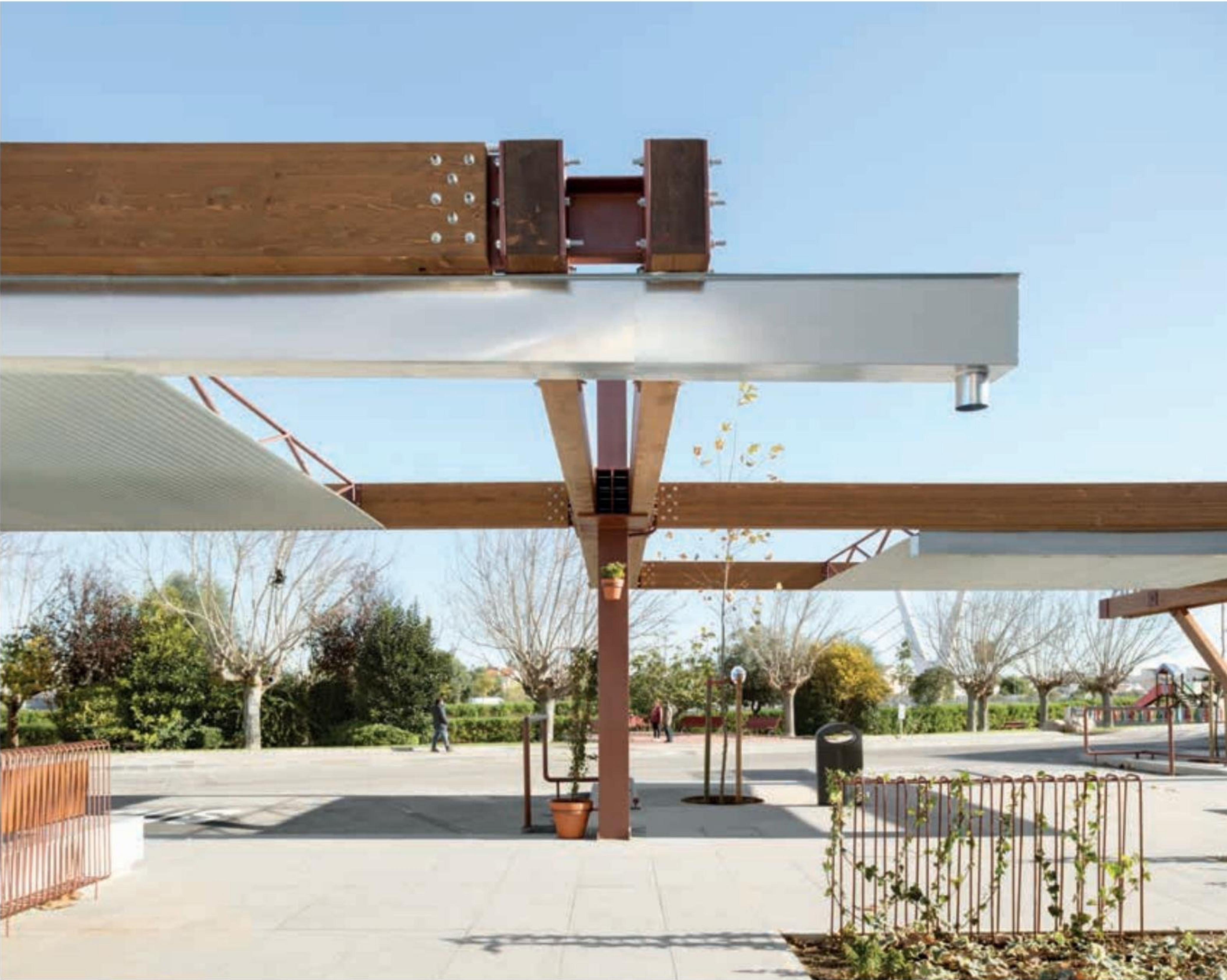
Square and bus stop in Vinaròs by Errería. Products by NAVARTI CERÁMICA.
